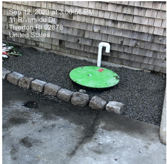
Figure 1 Typical grinder pump installation at surface.
